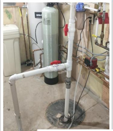
Sump Pump to Floor Drain
